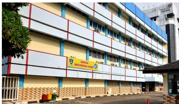
Building that houses the SMP and SMA St. Antonius.
